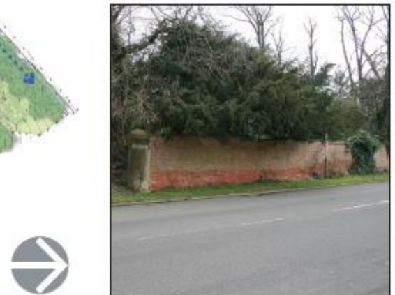
Existing Boundary Wall
