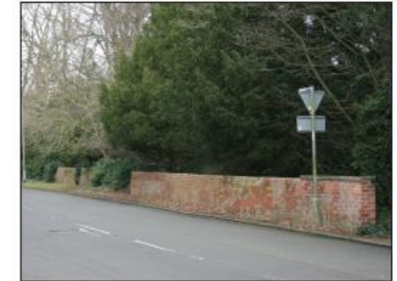
Existing Boundary Wall
