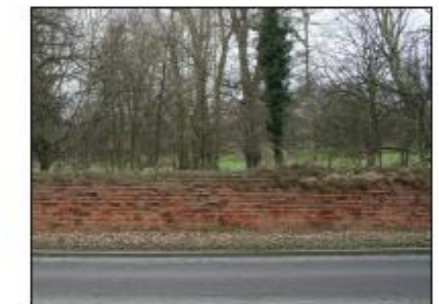
Existing Boundary Wall
